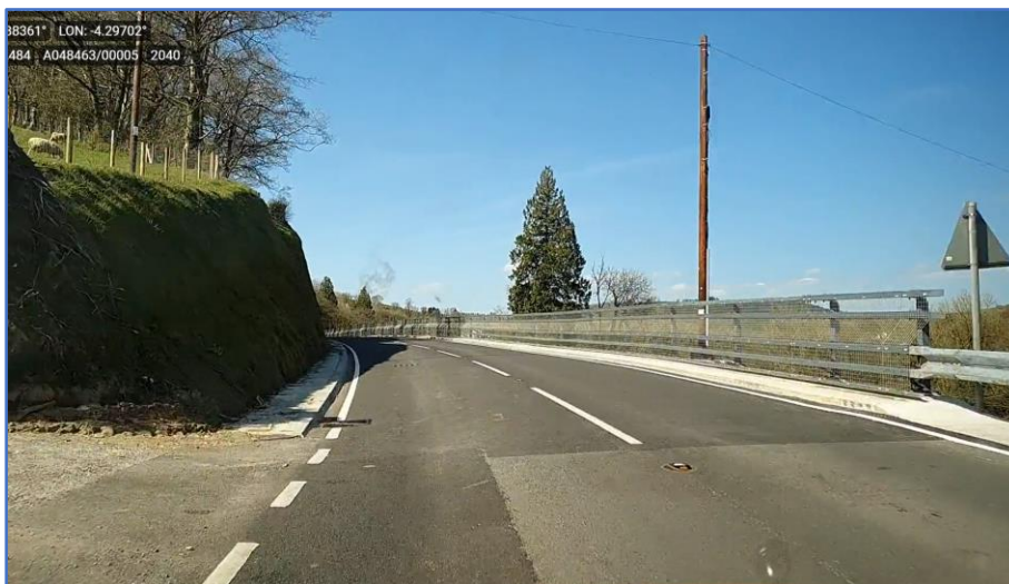
A484 Pante Retaining Wall
